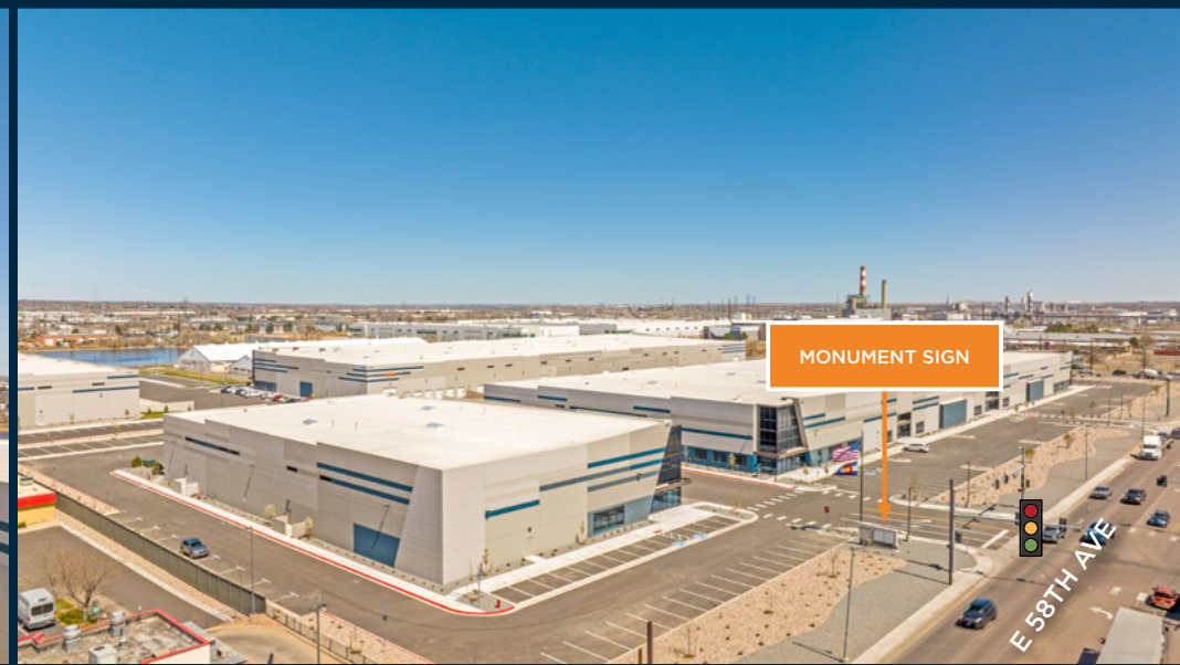
E. 58th Avenue Entrance with signaled entry and monument signage
